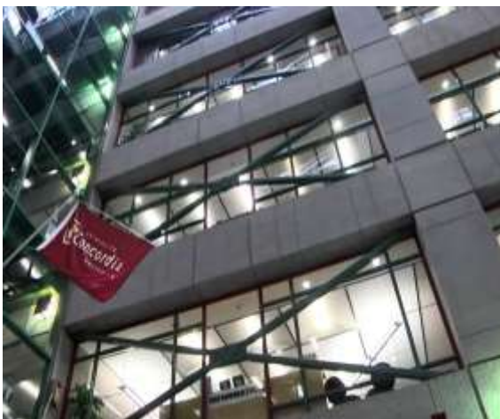
Fig.4:Friction damper in frame
