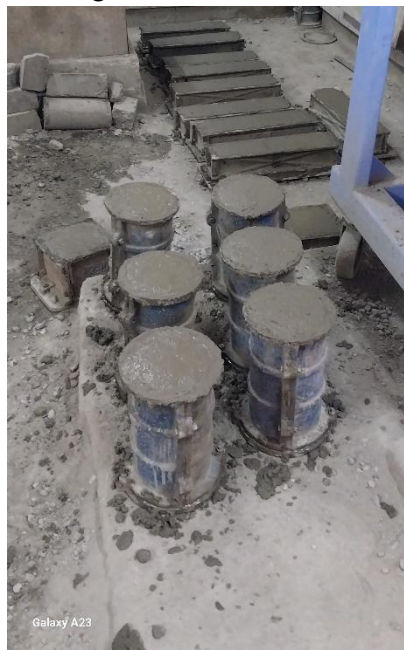
Figure1 (b)- Casting of Beam and cylinder specimen
