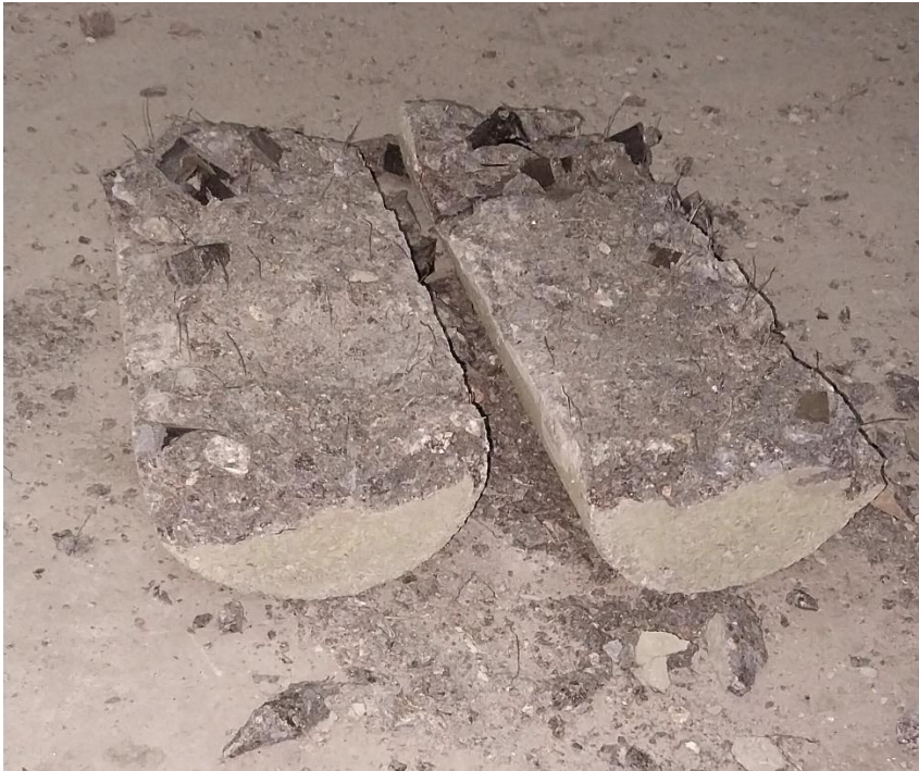
Figure 2-b: Steel fibers inside the concrete
