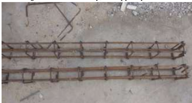
Fig. Steel Reinforcement for the beam
