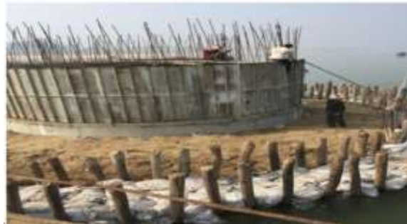
Fig. Construction of false Steining with cofferdam
